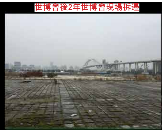
expo site demolition 2 years after Expo
